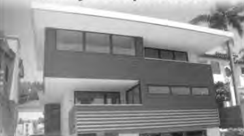
This remodeled Net Zero home has $0 electricity and gas bills.
